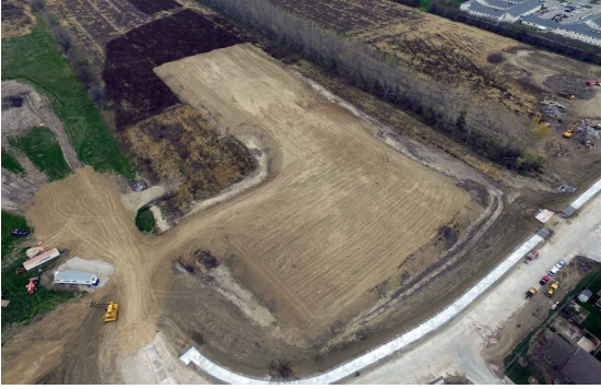
Surcharge improves and pre-compresses existing soils.
