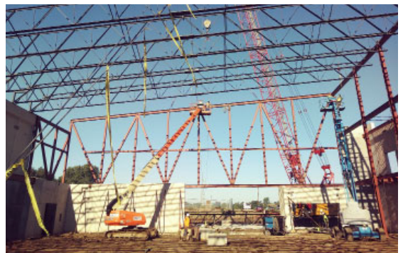
Tube steel truss.
