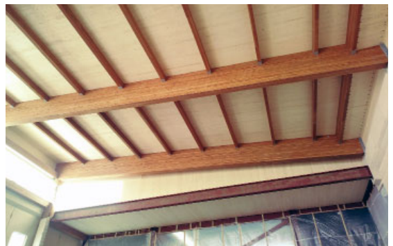
Interior ceilings combine glulam wood beams, wood decking, and stained wood soffit panels.
