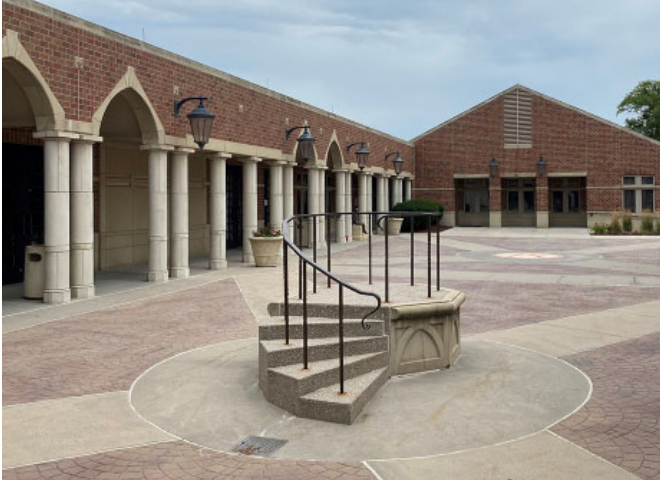
Exterior pulpit and courtyard entries to the Church and Parish offices.
