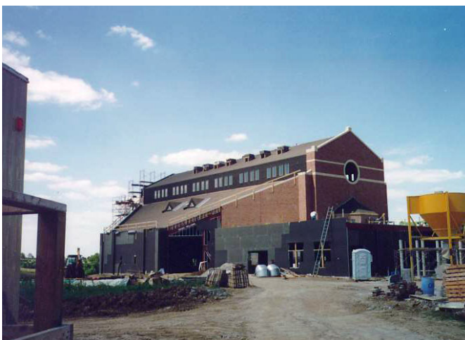
Photo courtesy of RDG. Phase III Sanctuary construction.
