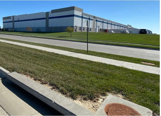
Building 1 from the parking area across Gold Coast Road.
