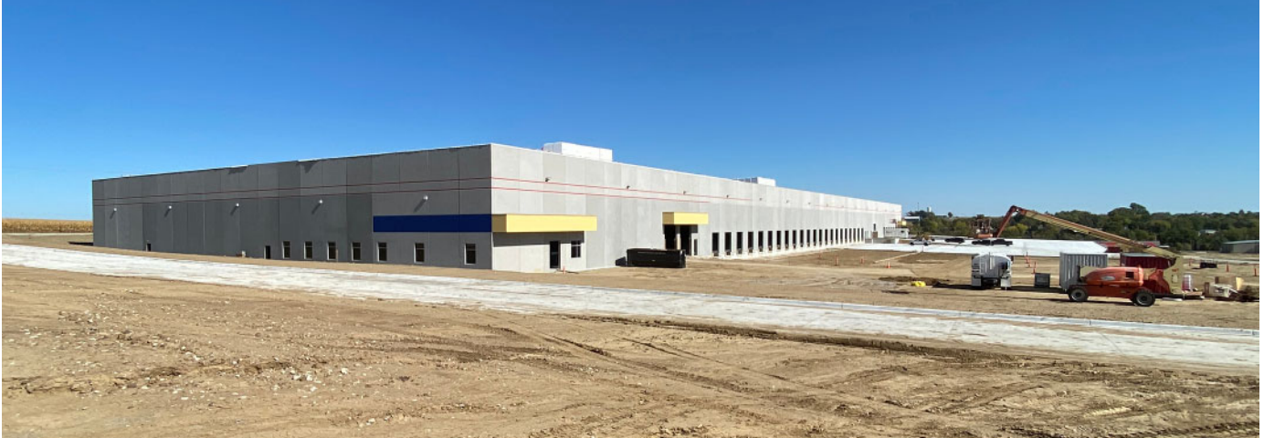
Springfield Commerce Building 1, Lot 1.
