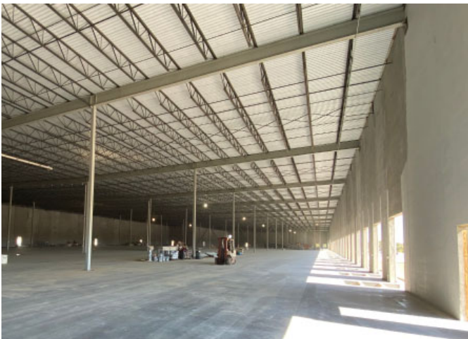
Steel deck roof, steel joists, steel beams, and steel columns.
