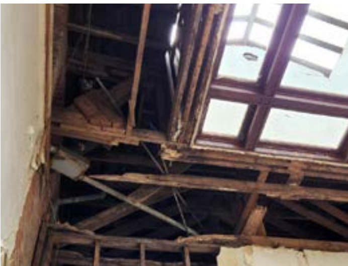
The deteriorated skylights and roof structure caused by years of moisture intrusion required extensive reconstruction. New wood framing members were installed to support the historic skylights.
