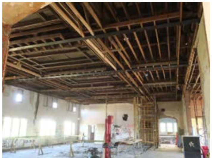
The deteriorated skylights and roof structure caused by years of moisture intrusion required extensive reconstruction. New wood framing members were installed to support the historic skylights.
